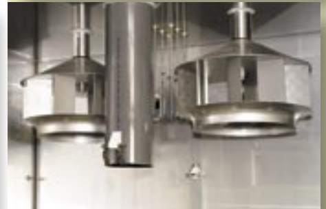
Hatcher fan units in stainless steel
